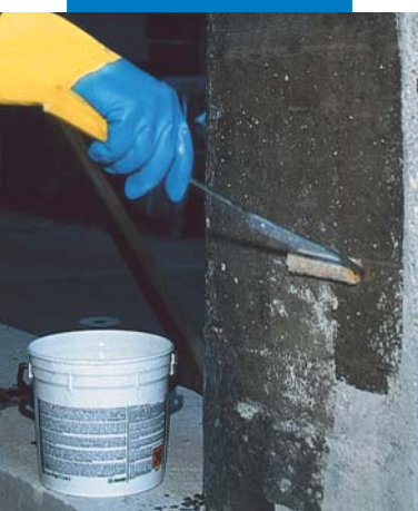
Applying a second coat of MapeWrap Primer 1
