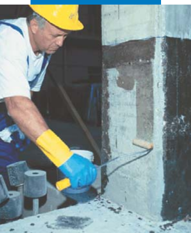
Applying a first coat of MapeWrap Primer 1
